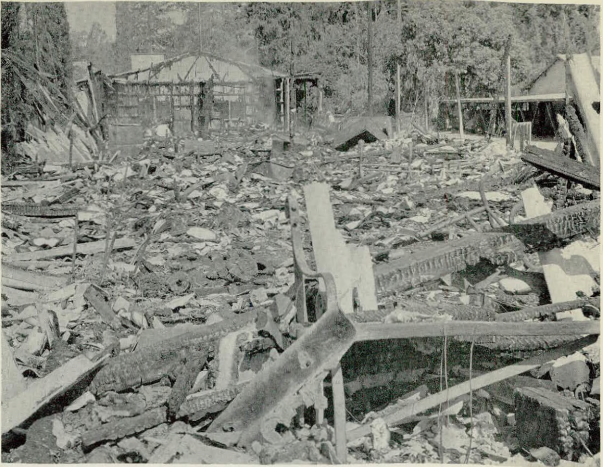
Remnants of the Water Resources, the Small Projects Planning Division and the Library of the Department. Forty years of drilling and hydrological records and some 7000 volumes of Library books have been destroyed by fire in July, 1974.
