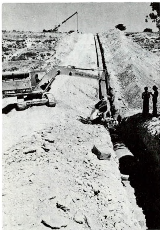
Installation of the western conveyor ductile iron pipes in progress.
