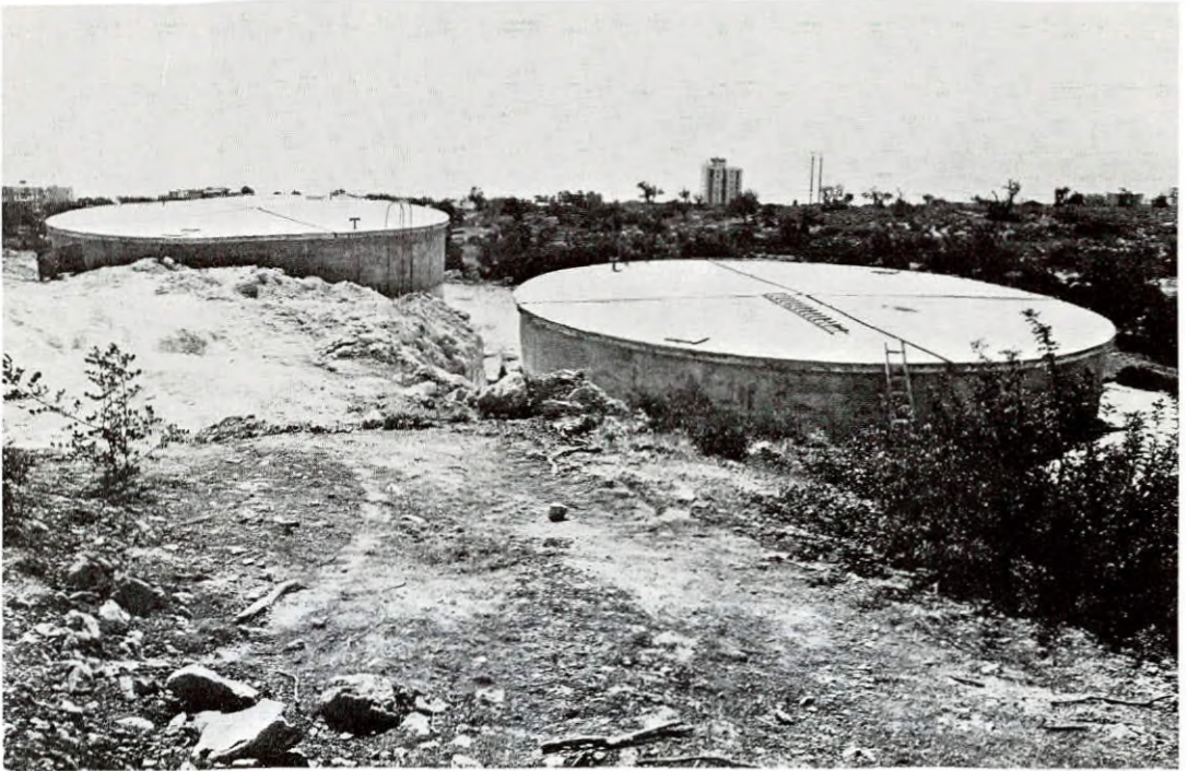
Amathus Improvement Board domestic water supply storage tanks of 1 000 m 3 total capacity.
