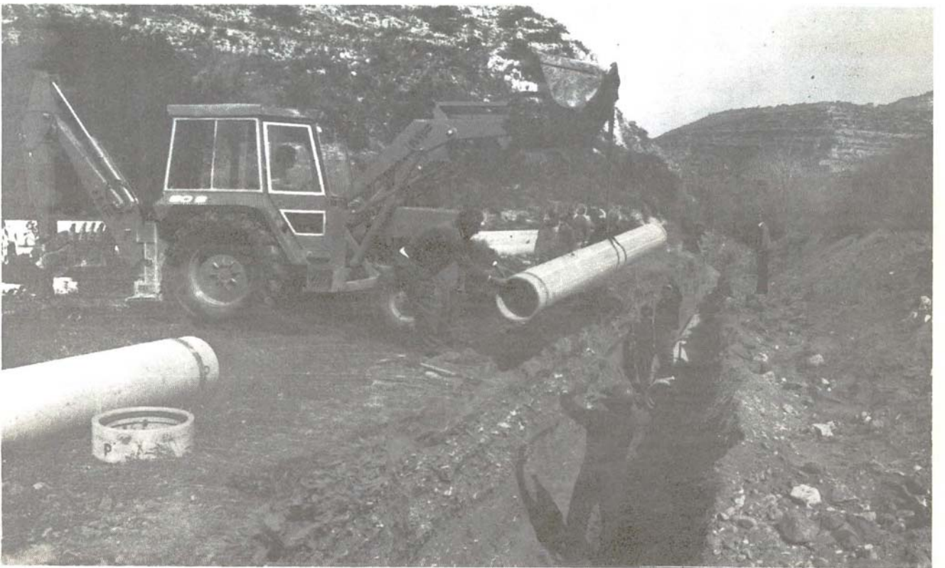
Pendaskinos Irrigation Area. Installation of pipes. WDD Photo B96EN-23A (13.3.85).
