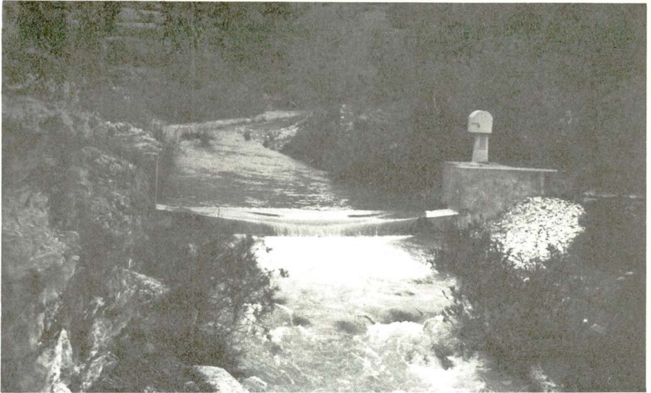
Flow gauging station at Kryos river near Khalasa measuring the inflow to Kouris Dam. WDD Photo B91EN19(18.2.85).
