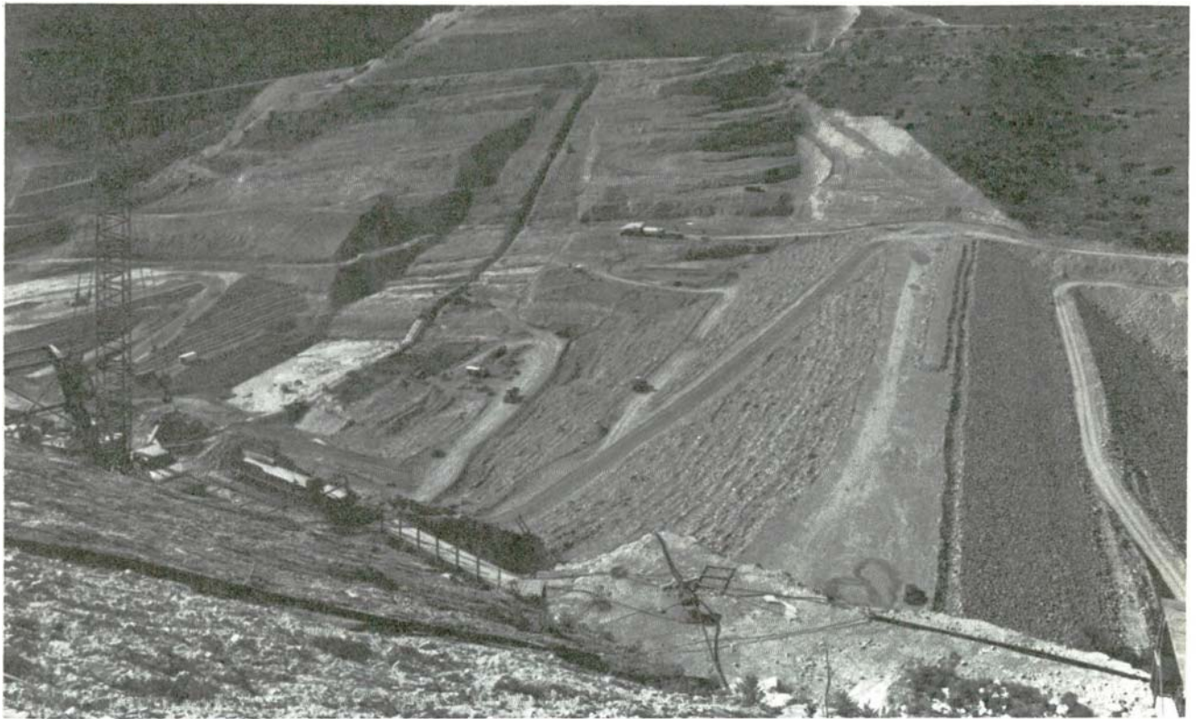
Kouris Dam under construction. WDD Photo C60EN-1(24.1.86)
