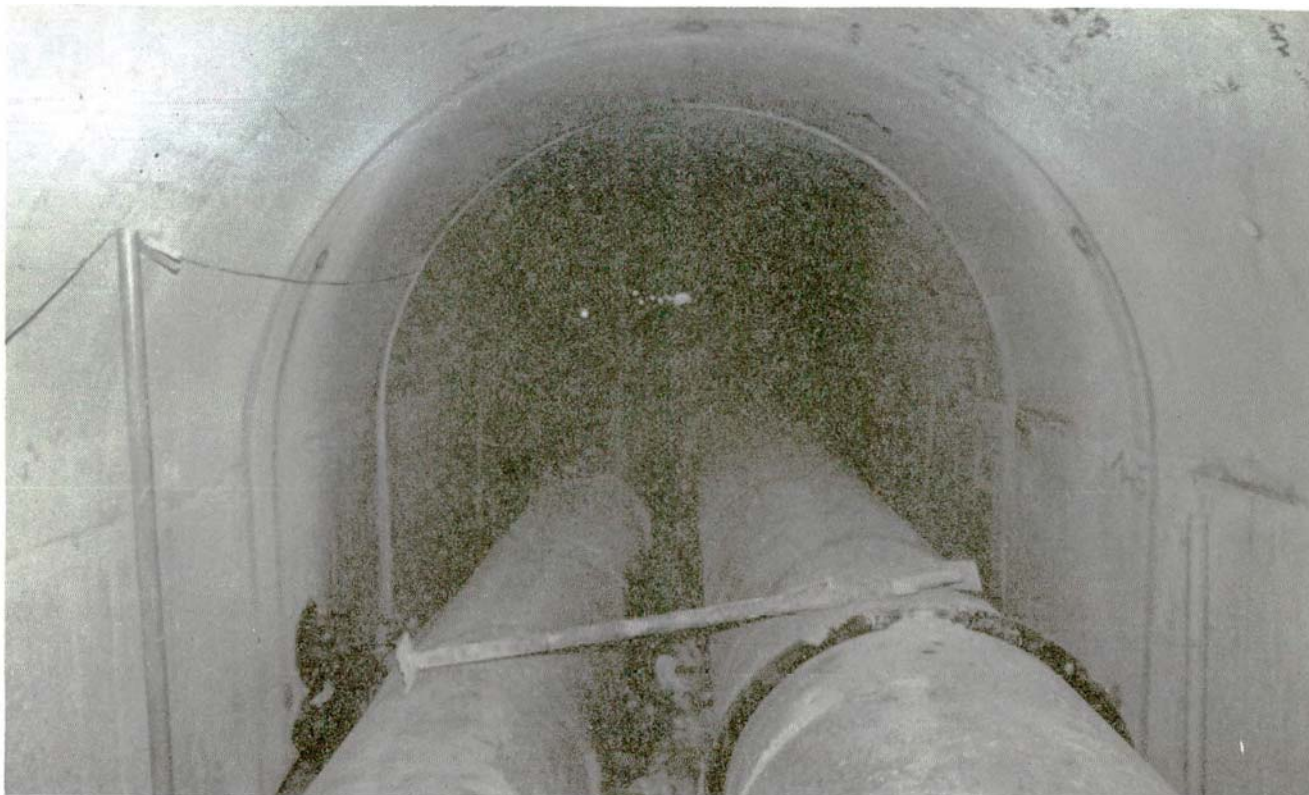
Evretou Dam: Outlet tunnel. WDD Photo C37 EN-15 (10.9.85)
