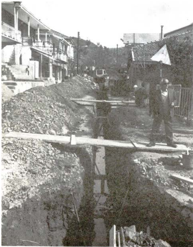
Kakopetria Sewerage Scheme. WDD Photo B99-EN-15 (26.3.85)
