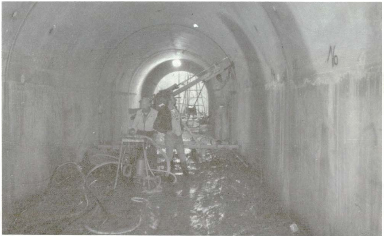
Evretou Dam: Drilling for tunnel consolidation grouting.
