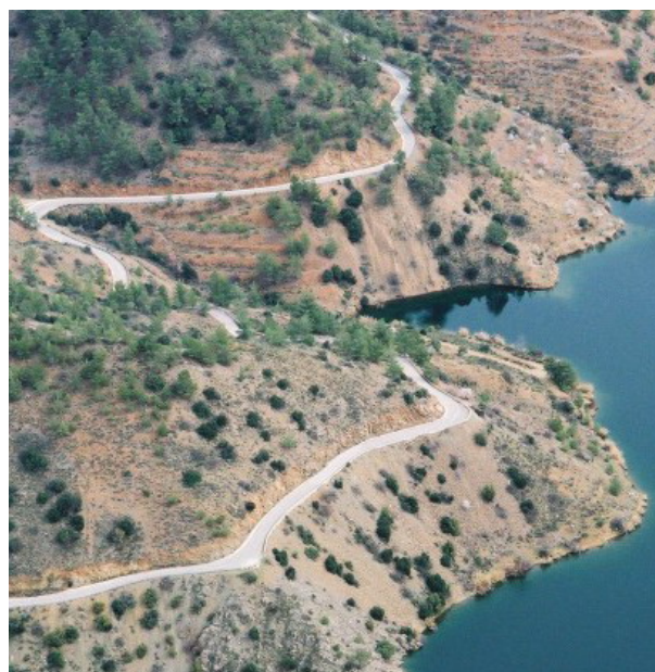
Example of “through traffic” road running along the bank of a dam lake (Palekhori dam - WDD photo). See also right bank of KOURIS dam at § 3.2.1
