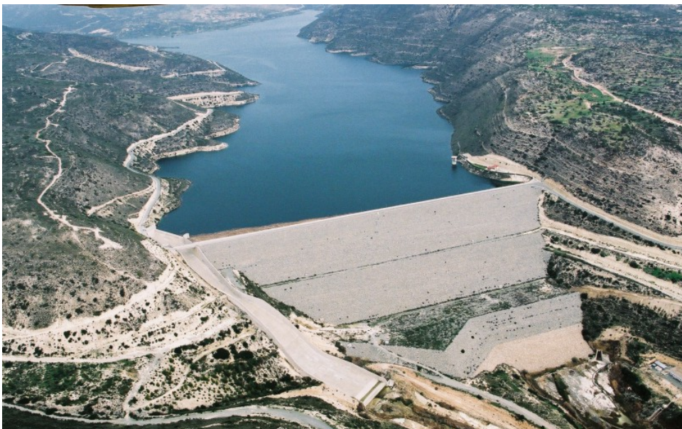
Kouris dam (WDD picture)
