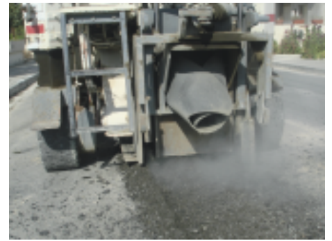
Cutting of asphalt
