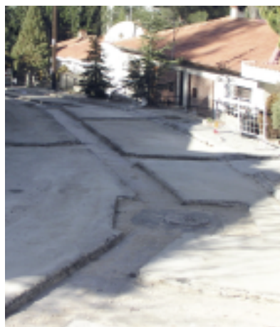
Laying of road base
