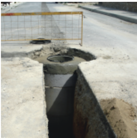
Construction of manhole
