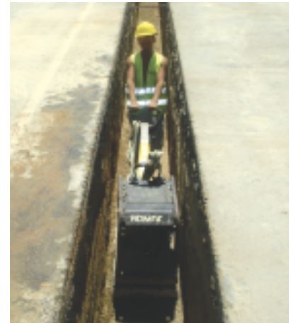
Compaction of backfill material
