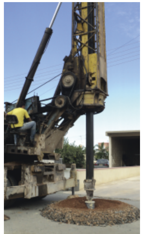
Drilling of manholes
