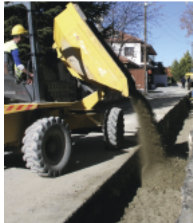
Laying of backfill material
