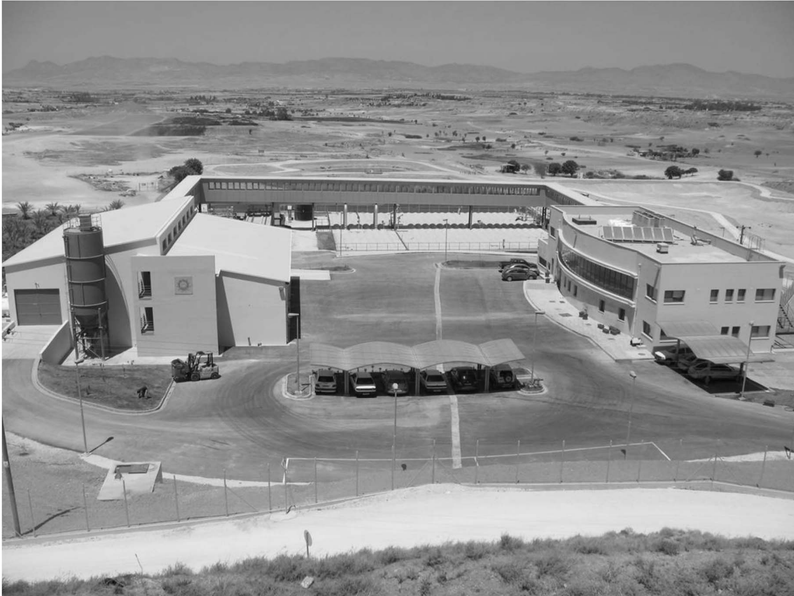
ANTHOUPOLIS WASTEWATER TREATMENT PLANT -SBN
