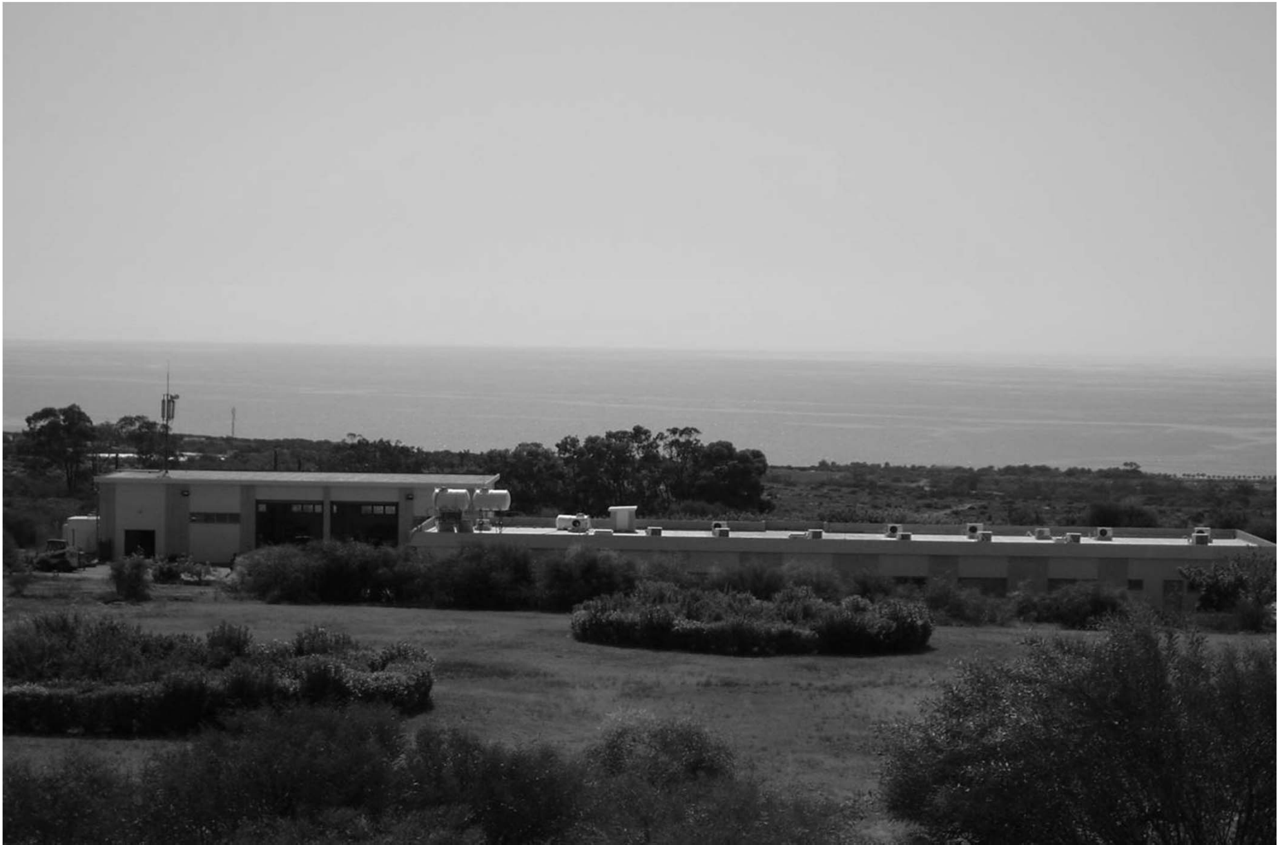
PARALIMNI-AYIA NAPA WASTEWATER TREATMENT PLANT
