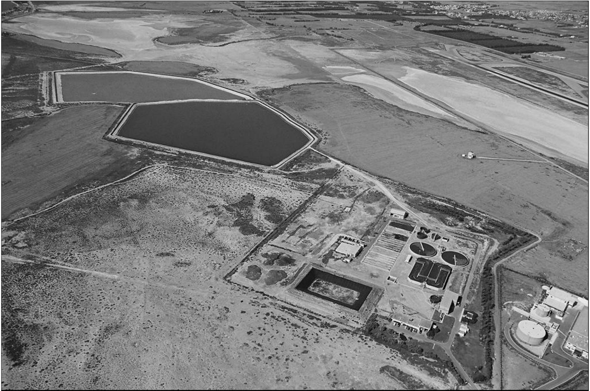
LARNACA WASTEWATER TREATMENT PLANT-SBL
