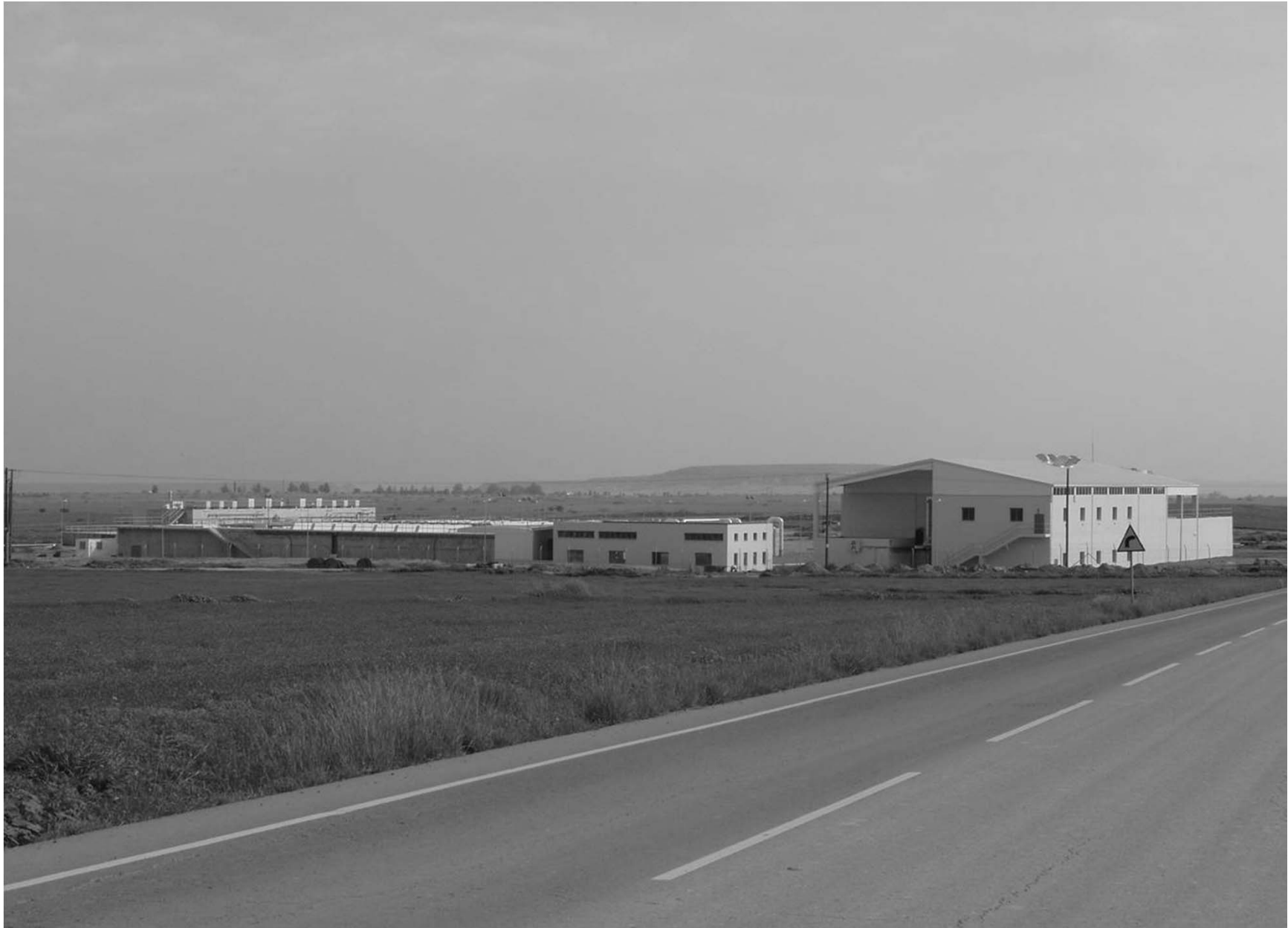
VATHIA GONIA WASTEWATER TREATMENT PLANT -SBN
