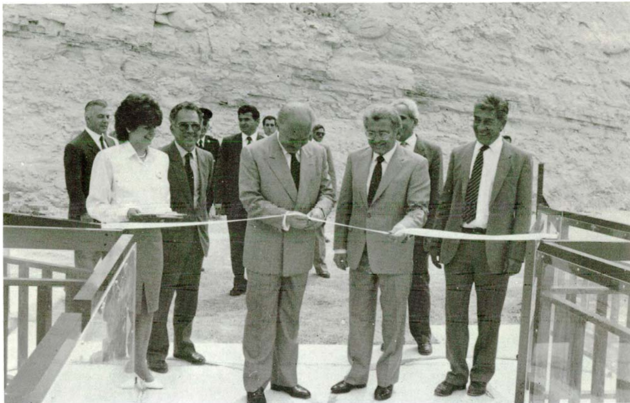
Southern Conveyor Project - Kouris Dam Inauguration of the Project by the President of the Republic Mr. G. Vassiliou on the 22nd of April 1989. The ceremony was attended by Members of the Council of Ministers, the Diplomatic Corp. and other officials.
