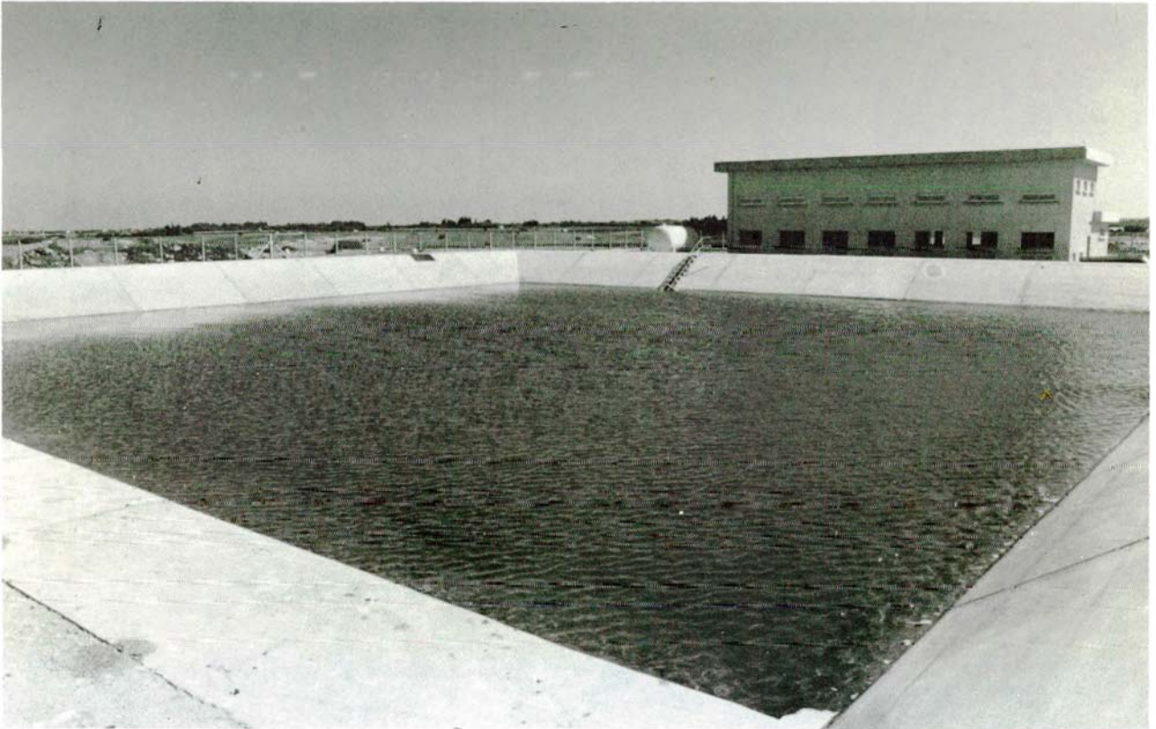
SCP-Kokkinokhoria Irrigation Area Central Distribution Point CDP XVI Pumping station and reservoir. WDD Photo G10EN-7 (10.10.89).
