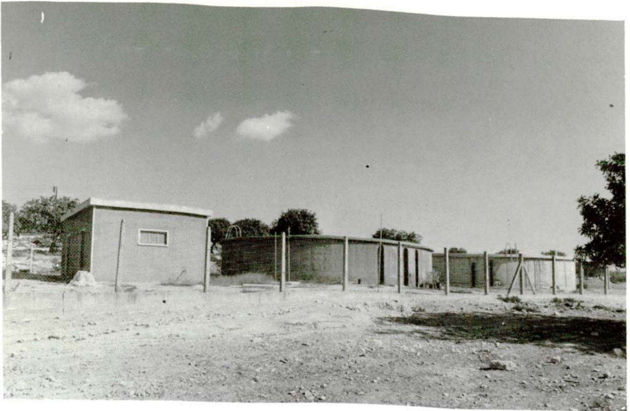
Erimi-Kolossi-Ypsonas Water Supply Scheme. Housing of the pumping station and reservoirs. WDD Photo G12EN-2 (12.10.89)
