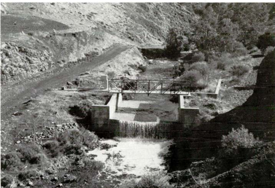
Flow gauging station on Ayios Onoufrios river near Kambia. WDD Photo No. F68EN-7 (12.1.89)
